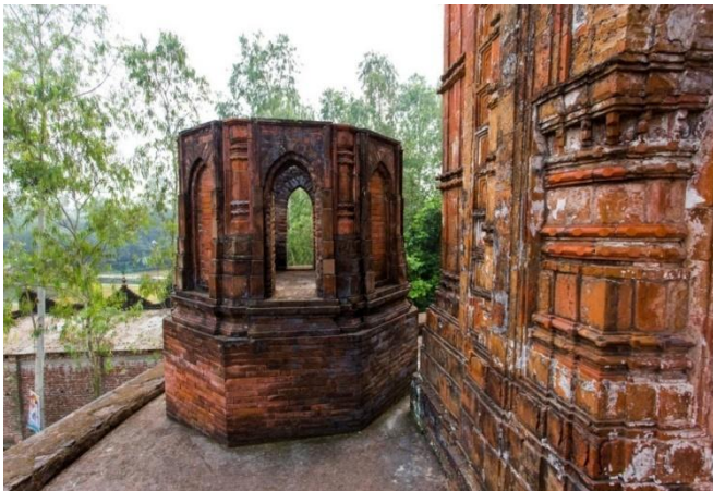
Fig. 9 Broken part of the dome of Nabaratna temple.
